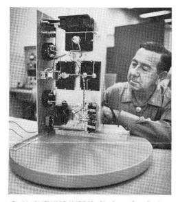
D. H. RUSHING (4213) displays the device he designed which serves as a rotating work table for checking electronic chassis. The device spins around like a lazy susan, allowing quick access to different sides.
